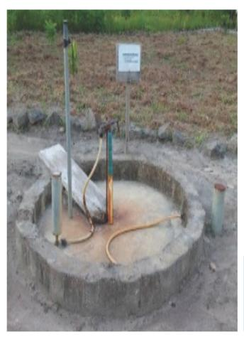
37mm to 50mm diameter, depth varies (7m to 100m— in fine sediment soil). Made from PVC pipes with couplings/other fittings, metal handle, filter material, timber footrest, and solvent with metal/timber pole for support when pumping.
